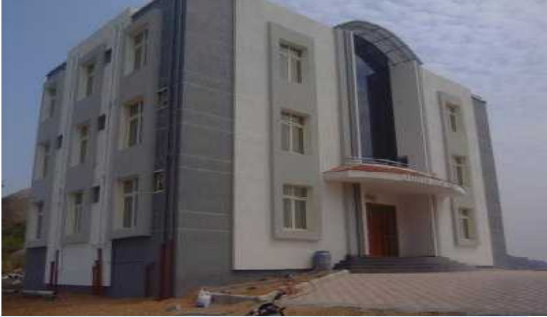
COMPLETED GUEST HOUSE BUILDING FOR SATAVAHANA UNIVERSITY AT KARIMNAGAR.
