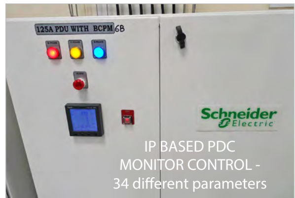
IP Based PDC Monitor
