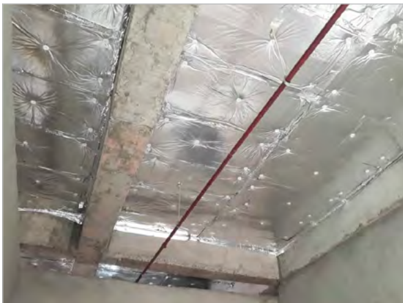
Thermal insulation System
