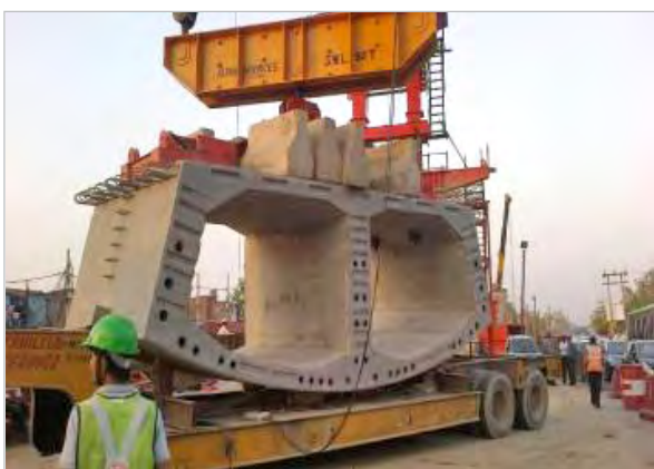
Fig. 5 : Transportation of Spine Segments
