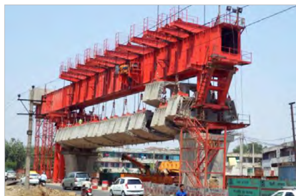
Fig. 6 : Erection of Spine Segments
